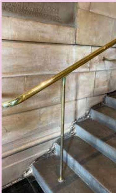
The stone stairs have brass handrails on both sides.
